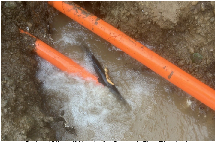
Broken 1" line off Monticello. Orange is Zipl Fiber boring into our black PVC pipe.
