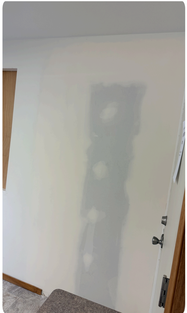
Picture of new wall in CWA main office
